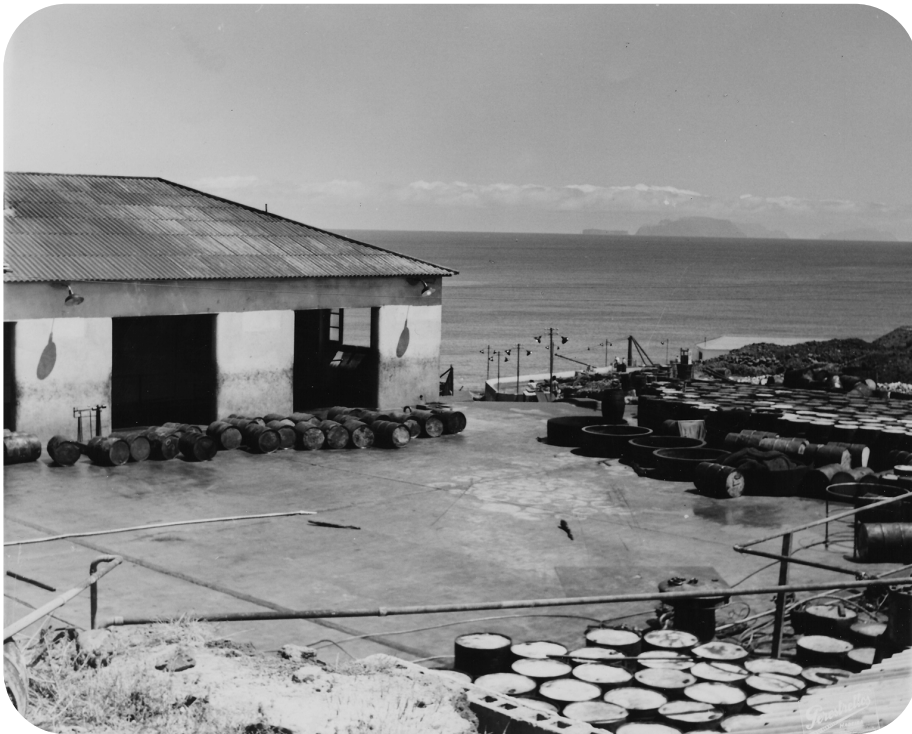
EBAM facilities, at Caniçal
